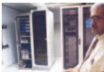
IT manager inspects ICASA main server room.
