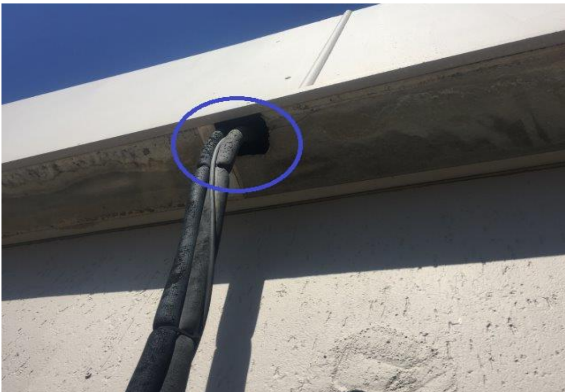
Cable Entry (existing air-conditioning pipe entry or equivalent can be used)
