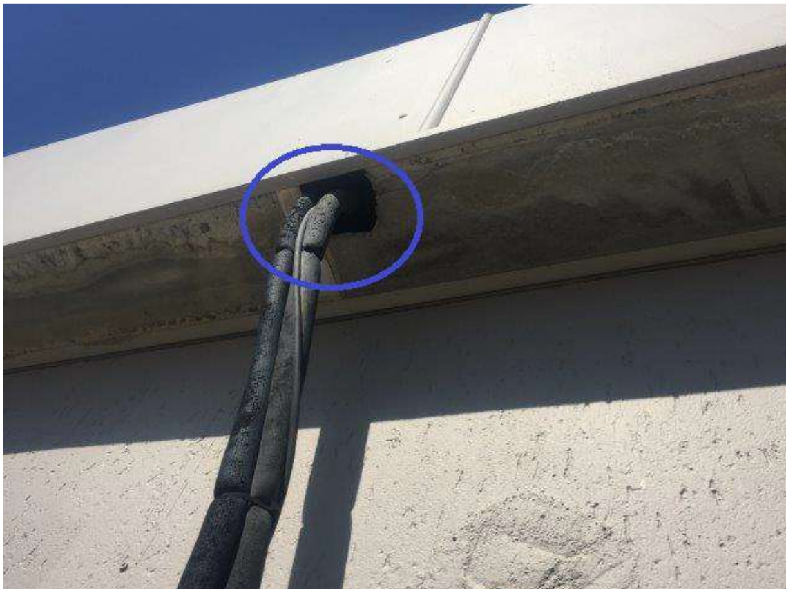
Cable Entry (existing air-conditioning pipe entry or equivalent can be used)
